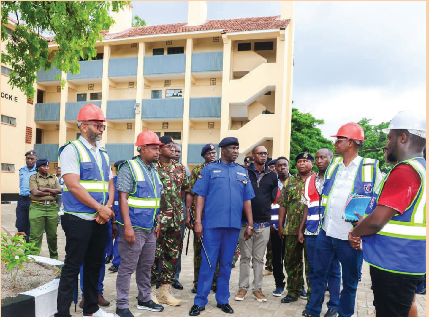
Inspector General of the National Police Service, Mr. Douglas Kanja, accompanied by senior officers, inspects the ongoing construction of the Telposta housing units in Makande and Bombolulu, Mombasa County, on 22nd April 2026.
